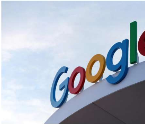
Google announced its new US$2 billion data centre in Malaysia had broken ground.
