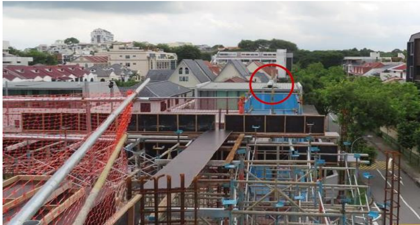
Construction of support structure
