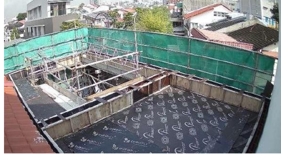
At the floor of a building under construction
