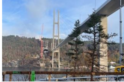
Highway - Norway Eiffage
