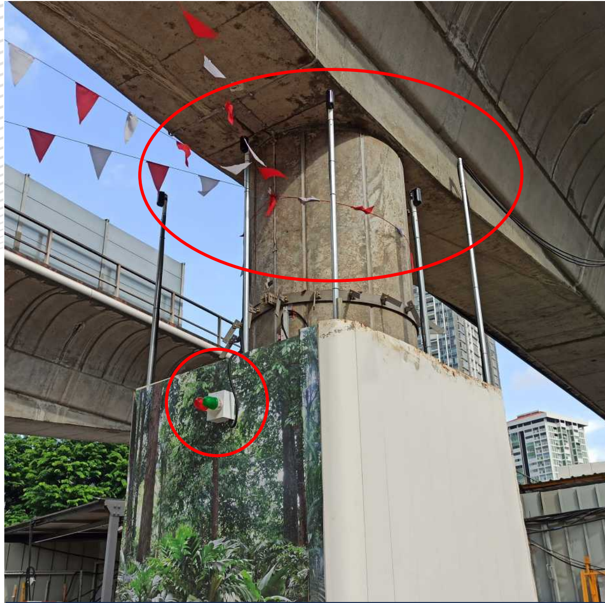
Photobeams located below MRT Viaduct at Jacking Shaft
