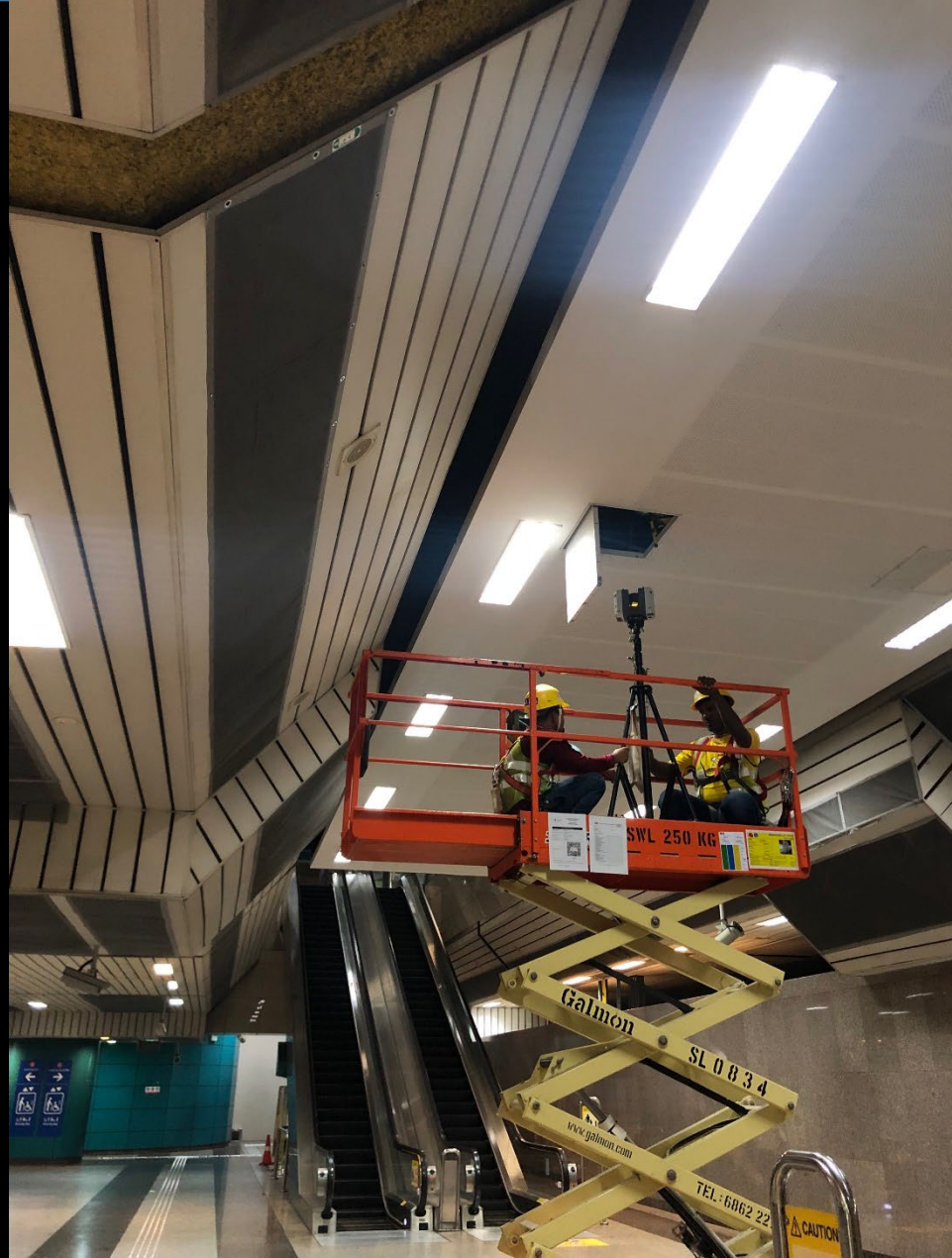
Leica 3D laser scan for BIM Model creation of Existing Station
