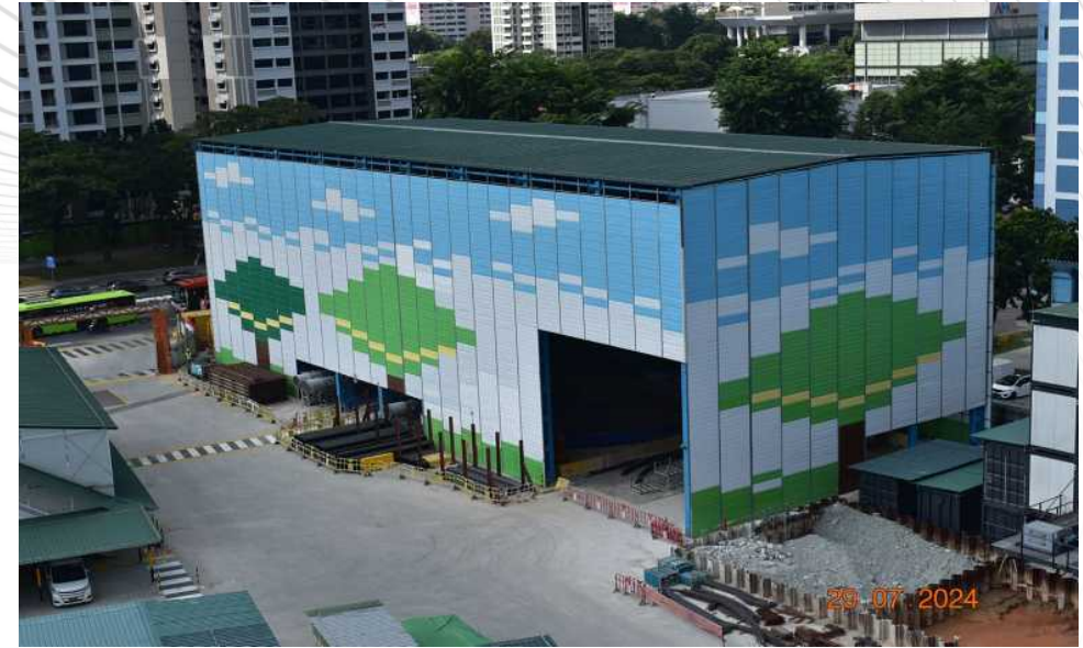
Full noise enclosure at launching shaft
