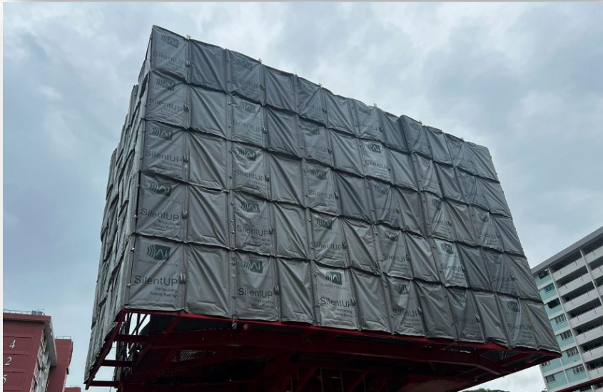
Silent Up install at machine
