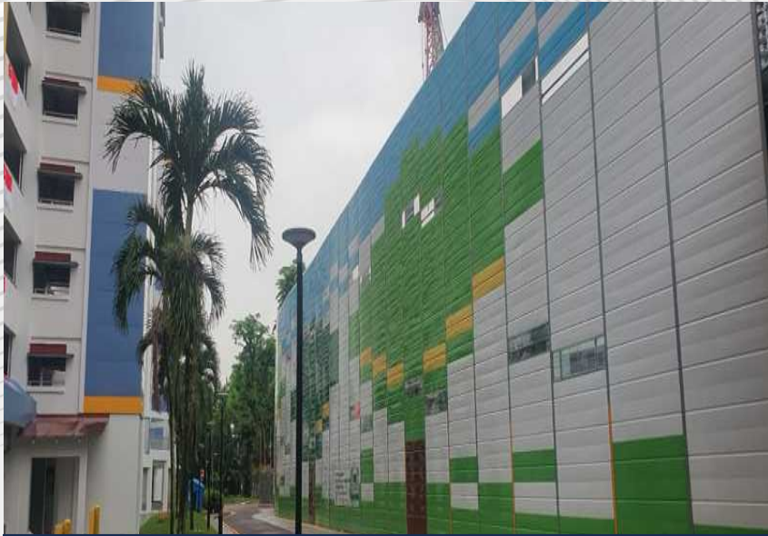
12m Noise barrier
