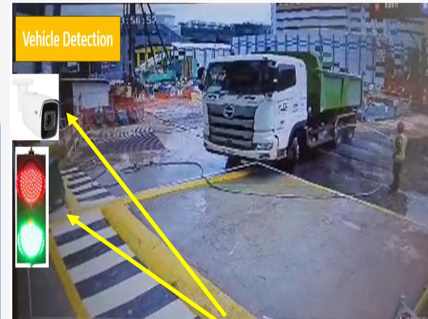
Internal AI Camera to detect vehicle & traffic light
