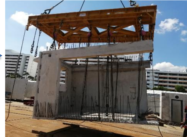
Lifted to check balance of the PPVC
