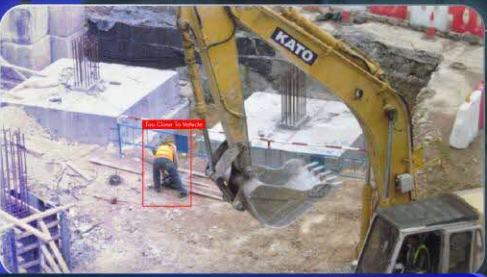
Workers near site vehicles
