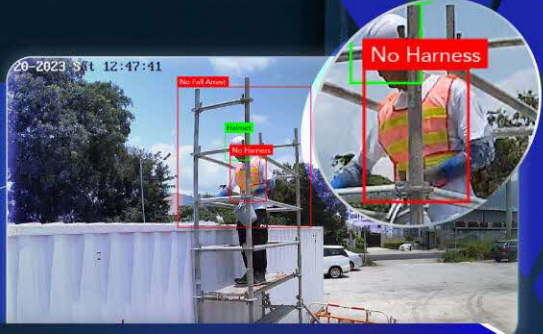
Working at height: No safety harness
